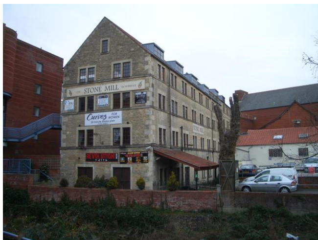
Stone Mills Main Building 2013
