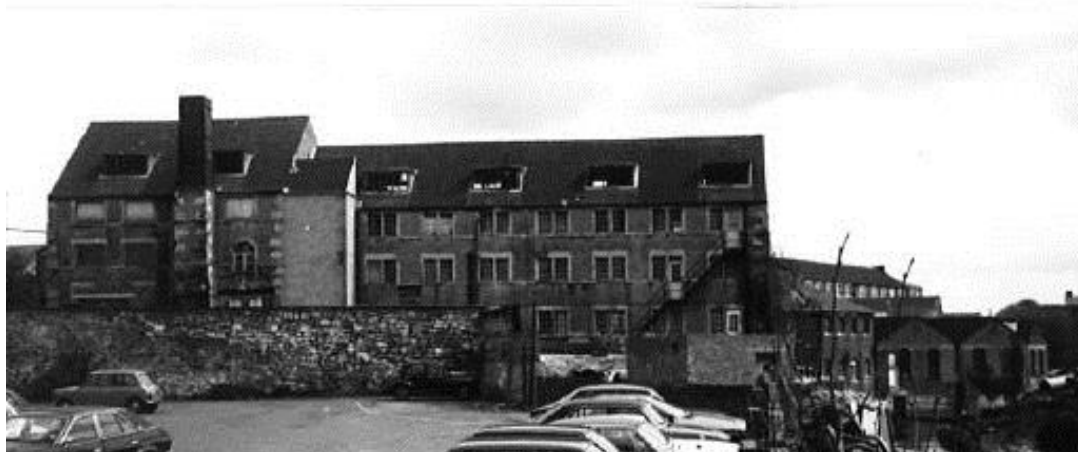
Main Building and Engine House 1980's from West.
